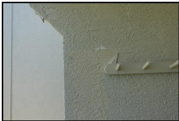
Figure 1 – Peeling and Faded Paint
