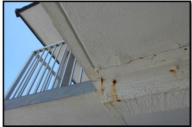
Figure 4 – Metal Support Corrosion
