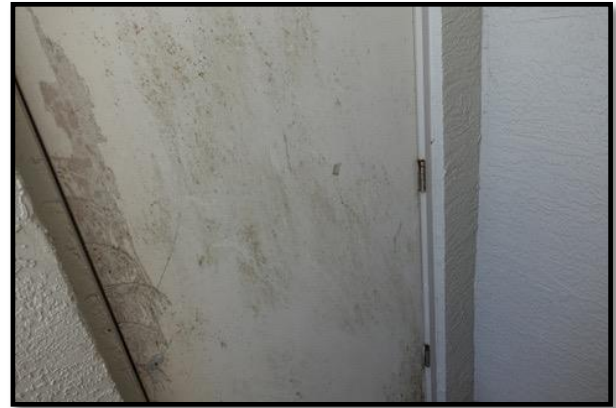
Figure 2 – Poor Door Finish
