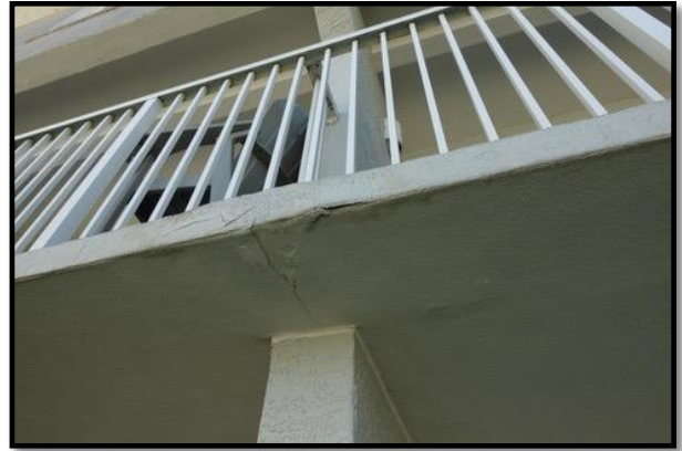
Figure 4 – Balcony Cracks
