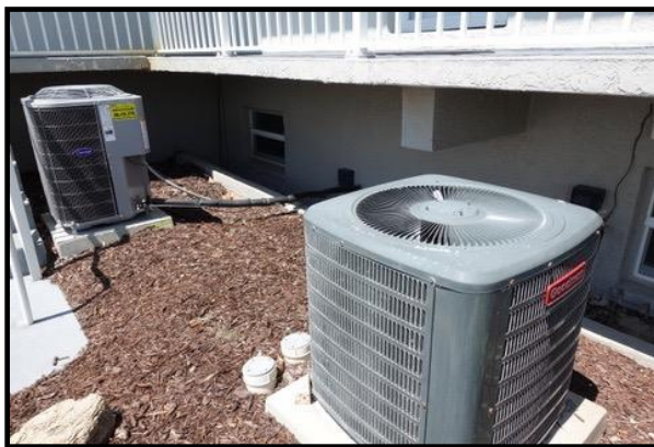
Figure 1 – Condensing Units
