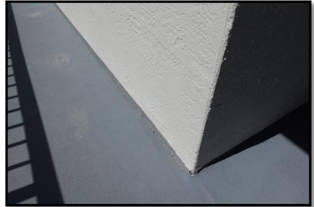
Figure 2 – Cracked Wall to Floor Seal
