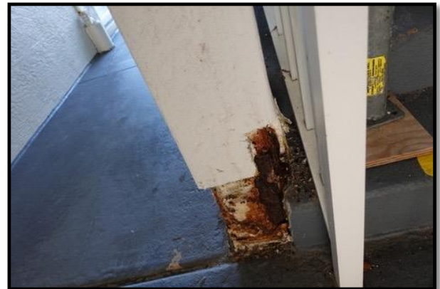
Figure 2 – Staircase Column Corrosion
