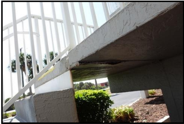
Figure 3 – Metal Support Corrosion
