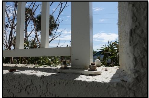
Figure 4 – Fastener Caps Missing
