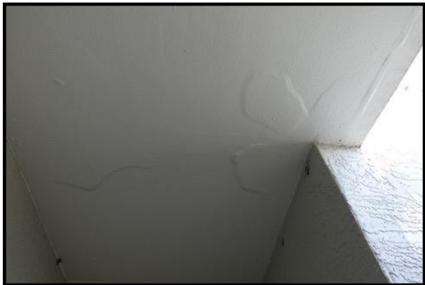
Figure 1 – Breezeway Side Ceiling Delamination
