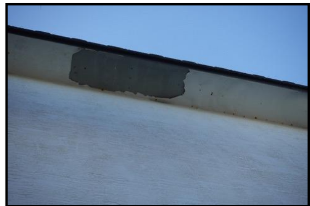
Figure 2 – Chipped Soffit Paint
