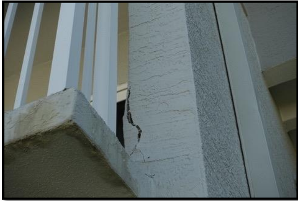
Figure 3 – Significant Wall Crack
