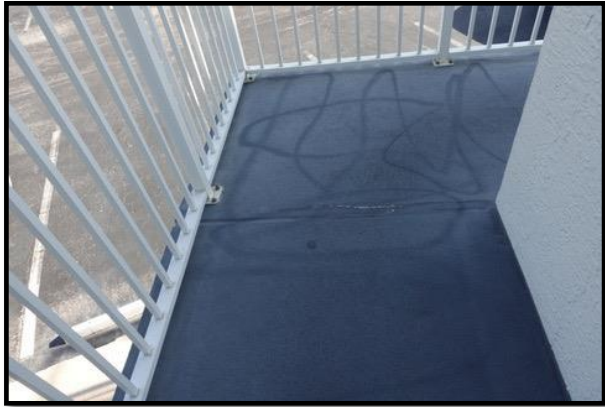
Figure 1 – Surface Crack
